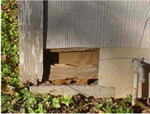
Various damaged areas missing siding and water damage noted.
