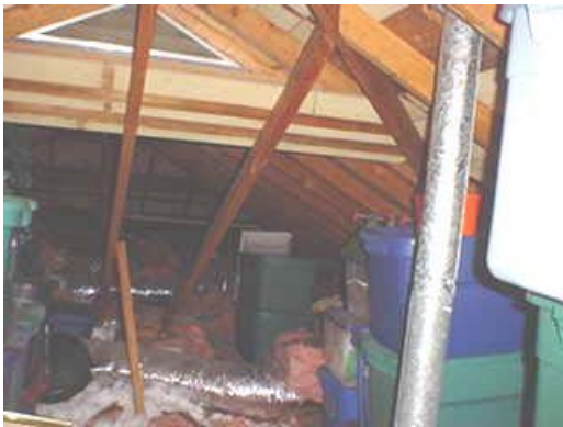
Recommend the addition of purlin roof rafter supports for the right side of back roof.
