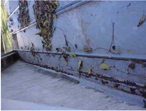
Vulnerable area where flat roof meets gable area.
