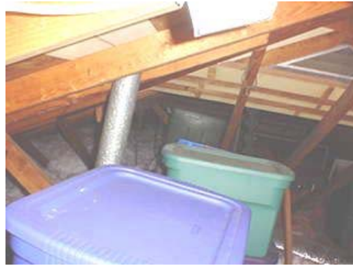
Recommend the addition of one more purlin stud support for the left side of the roof structure.
