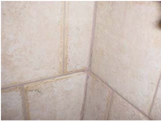
Re-grout and caulk corner in the main bathroom.
