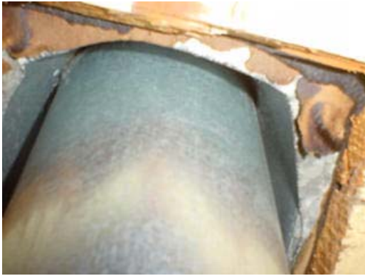
Note paper that shows burn marks from heater flue vent.
