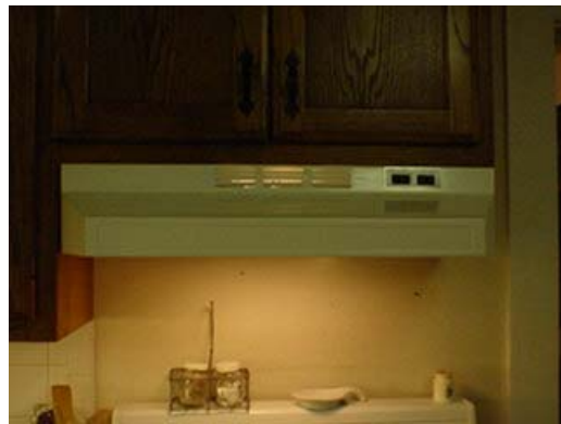
With the use of a gas stove the vent should be vented to the outside. This unit is a re-circulation vent hood.
