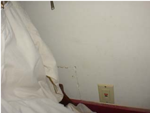
Access panel for whirlpool pump, GFCI protection for pump, located in master closet.
