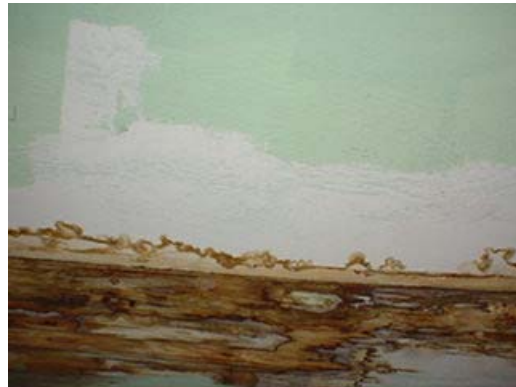
Evidence of several areas that leak by numerous water damage locations throughout the garage, washroom and carport areas.
