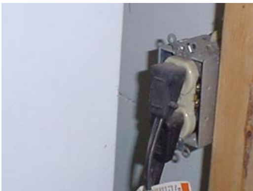
Electrical receptacle cover missing.
