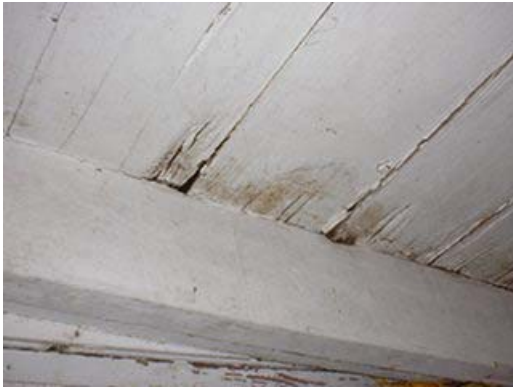
Water damage to decking located on flat roof over carport.
