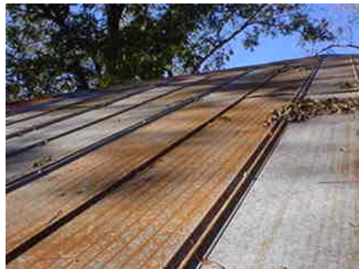
Areas of rusted metal roof material.
