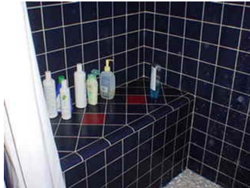
Shower stall seating area vulnerable to leaks, Monitor this area and re-grout and re-caulk as needed.
