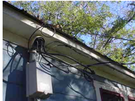
Electrical service wiring entrance too low by today's standards. Should be repaired.
