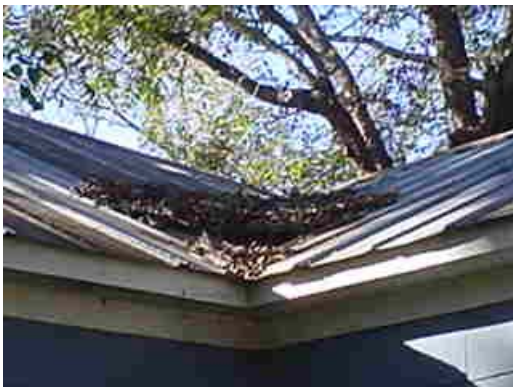
Suspected cause of concern is the two-pitched areas that meets and forms a flat dead valley area, which can collect water.
