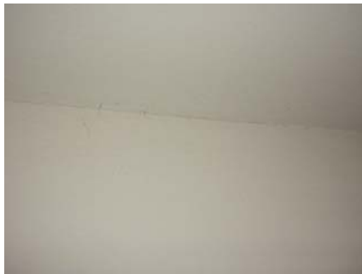
Small cracking observed where wall and ceiling meet - master bedroom.
