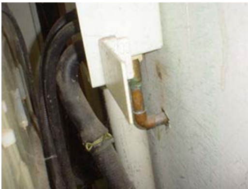
Water pipes too exterior wall should be insulated.
