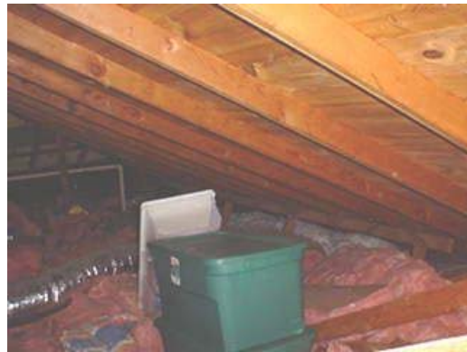
Recommend purlin roof rafter supports added here.
