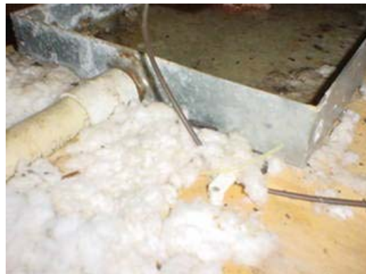
Standing water in overflow pan should be further investigated/ possible clogged main drain
