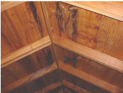
Ridge board considered being of insufficient size.
